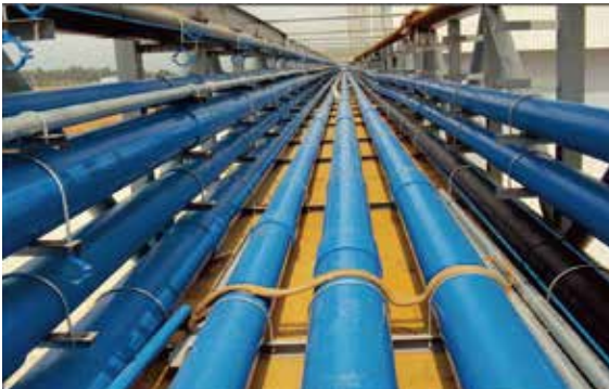
Water supply and drainage pipeline 給排水工程管道
